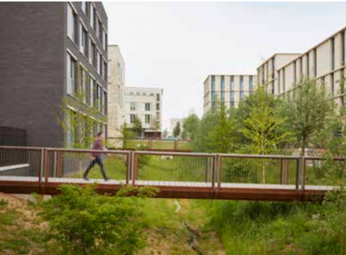
Fig.20: Bio-swale integrated into North West Cambridge campus
