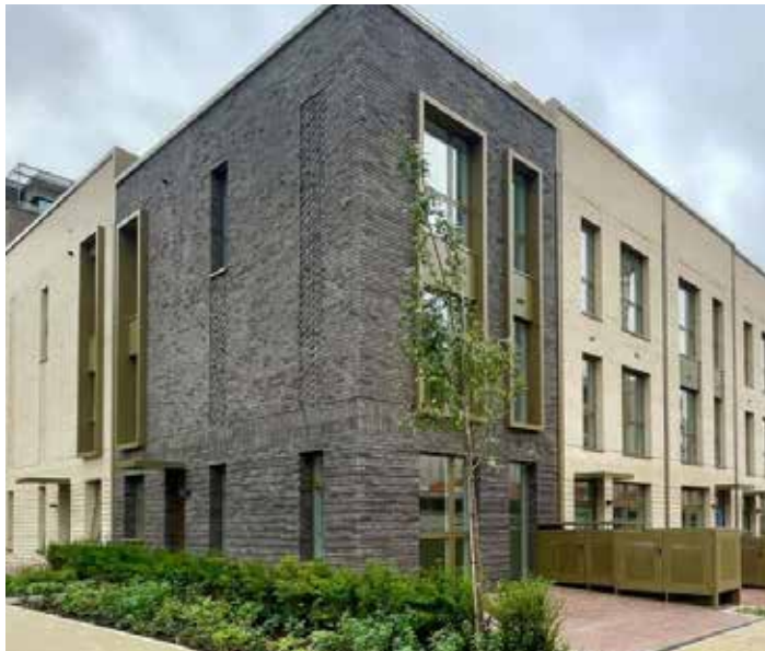
Fig.43: Corner building, Kidbrooke Village, London
